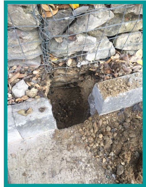
Foundations are dug
