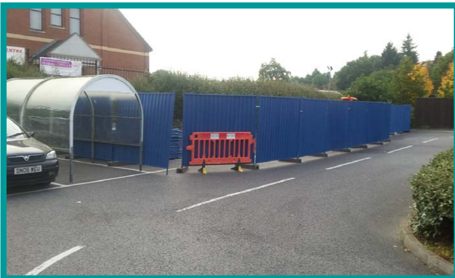
Area of installation is sealed off
