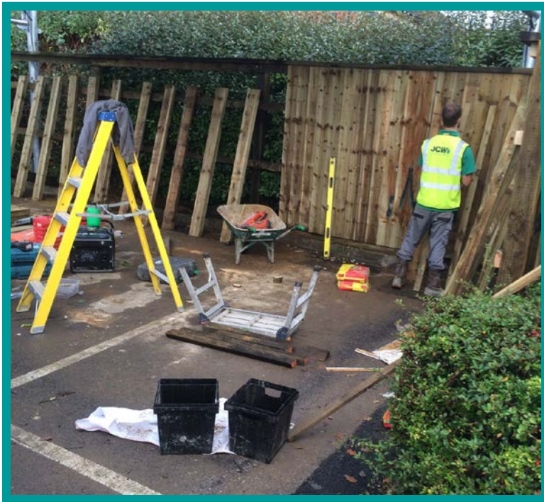
Erecting the fence
