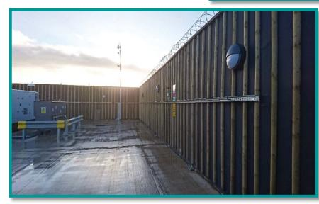
The JCW Absorbent Sound Screen conforms and tested to BS EN 1793. Also tested and complies to BS EN 1794-1 and BS EN 1794-2.
