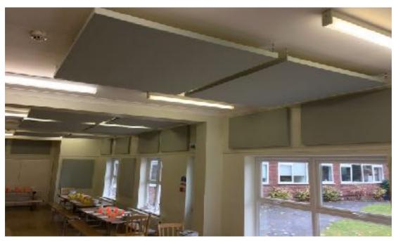
As JCW Acoustic Supplies Ltd can offer bespoke sizes of panels in different colours, we used different sizes of panels to suit the required amount of absorption needed and our expert installation team had no problem fitting these in over a two day period.
