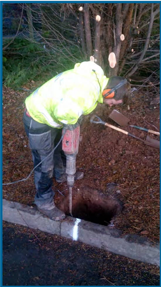
Digging the foundations
